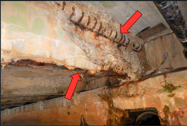
GIRDER 2S NEAR EAST ABUTMENT
