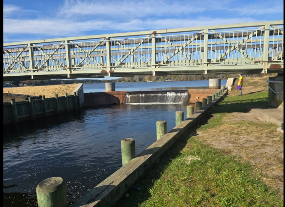
PEDESTRIAN BRIDGE NORTH OF STRUCTURE
