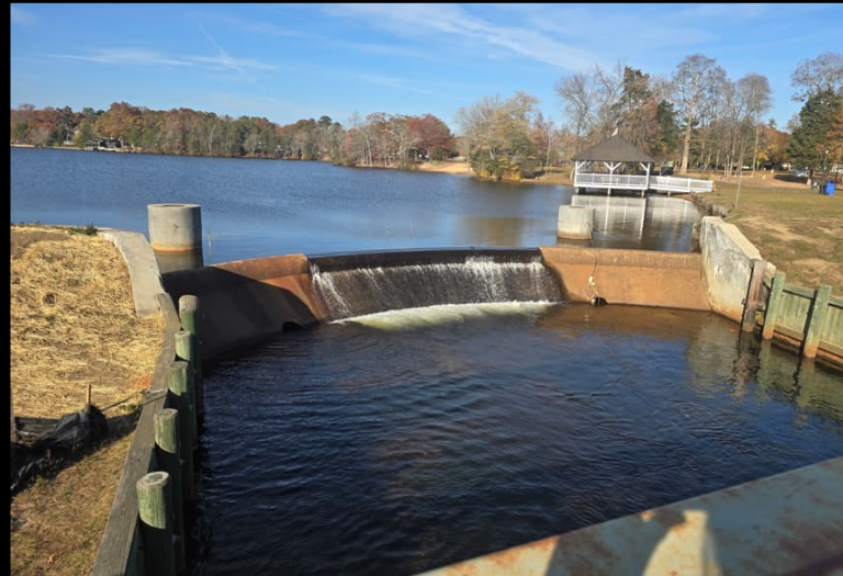
SPILLWAY LOOKING NORTH
