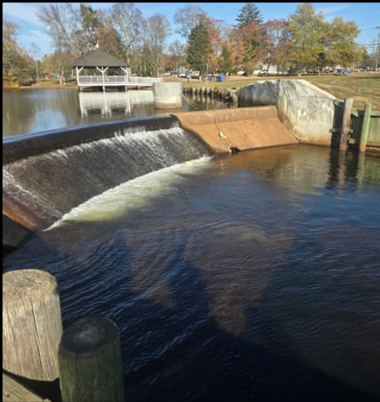
SPILLWAY LOOKING NORTHEAST
