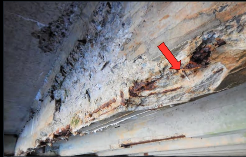
NORTH FACE OF GIRDER 11S
