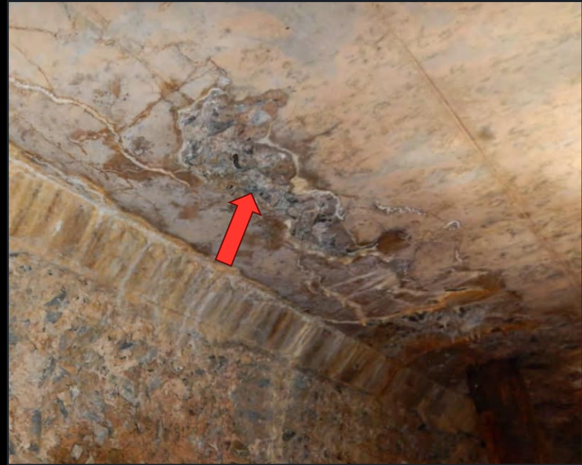
UNDERSIDE OF DECK BAY 2S
