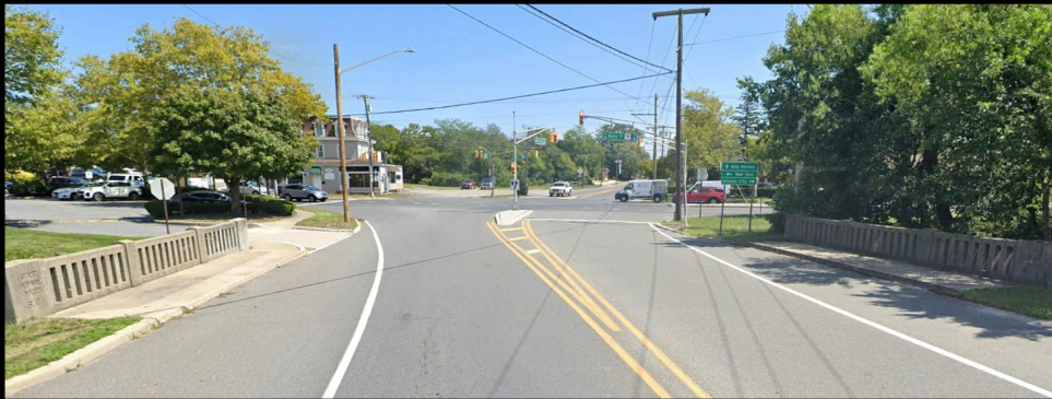
WEST APPROACH LOOKING EAST
